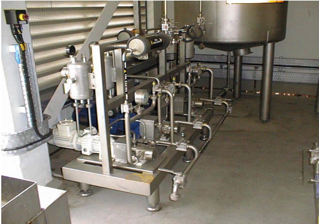
FIGURE 3: EXAMPLE OF ENZYME TRANSFER PUMP SETS
